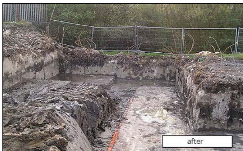
Same area after remediation
